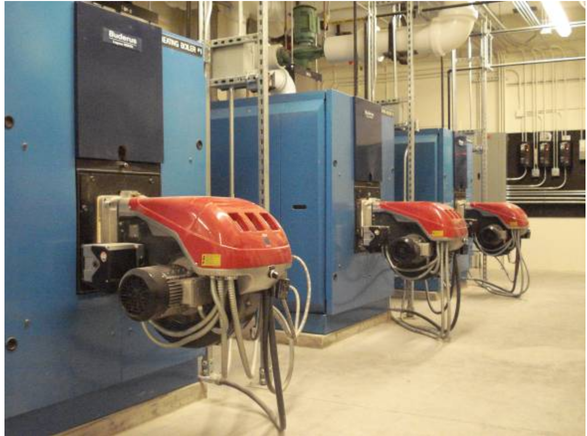
G615 Commercial with Riello Burners Application: a New England High School
